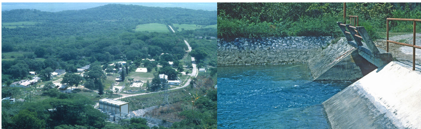
Left: view of the hydroelectric plant complex on Rio Salto above the cascade. The plant generates electrical power for residents and commercial enterprises such as sugarcane mills. Right: section of construction to re-direct Rio Salto into large conduits to feed the hydroelectric plant. Aug. 1981.
